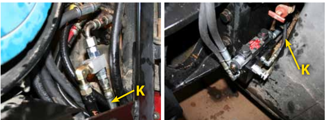
Figure 1-11: Install Pressure, Tank and Load Sense Hoses
