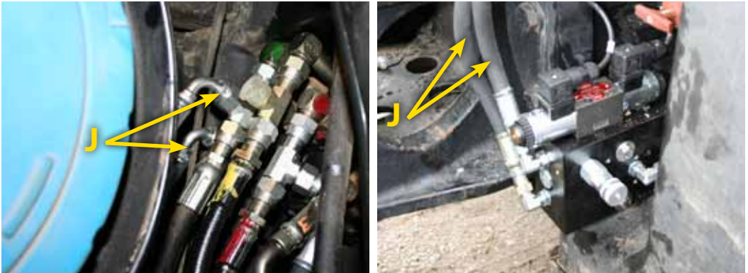
Figure 1-10: Install Pressure, Tank and Load Sense Hoses
